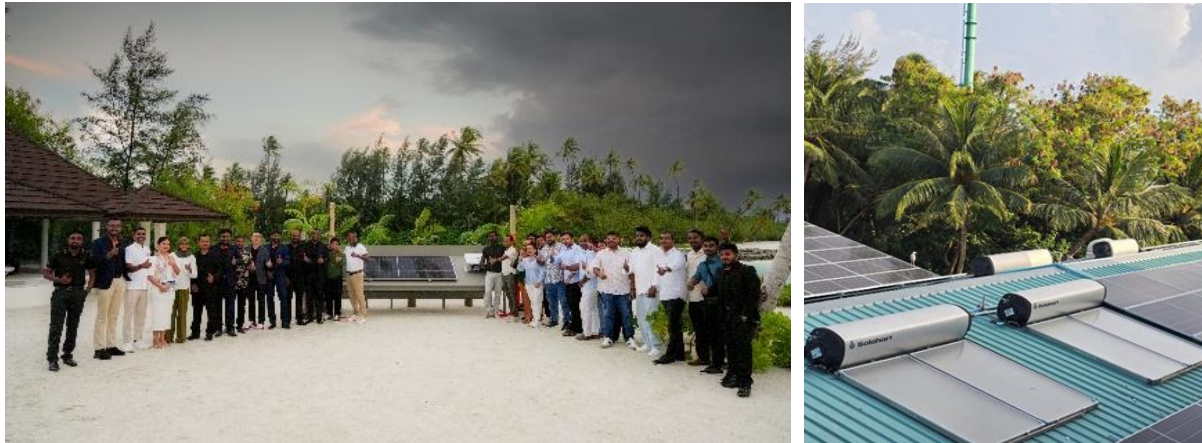
Best Practices 1- Laundry Hot Water Usage Generate from Solar Hot Water System
